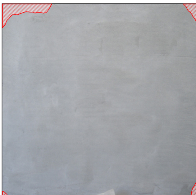
図-3.2.23 No.1 浮き・ひび割れ発生状況[P1]
