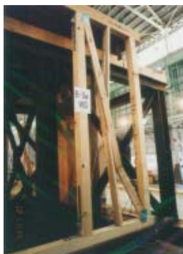
写真3, 筋かいは座屈 (LVL筋かい) Backling of Brace using LVL
