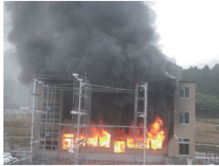
Photo 12: Fire spreads to the second floor (83 minutes after ignition)
