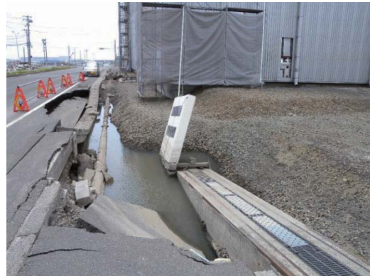
Photo 9.2-9 Excavation of ground
