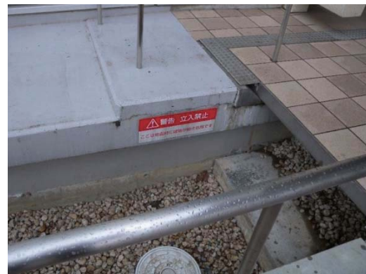
(b) Sign board to warn about seismic gap
