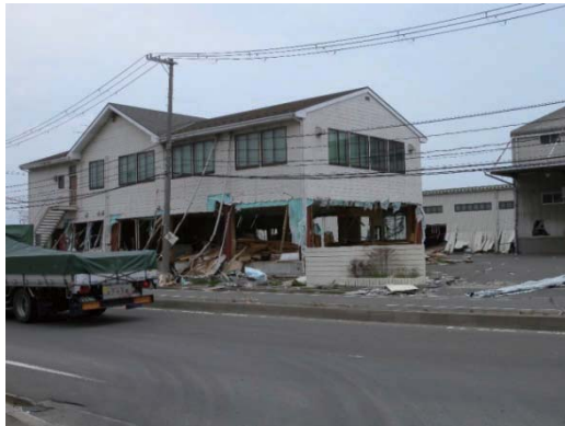
Photo 9.2-8 Tsunami damage to surrounding buildings
