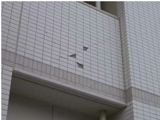
Photo 9.2-13 Drop of ceramic tiles
