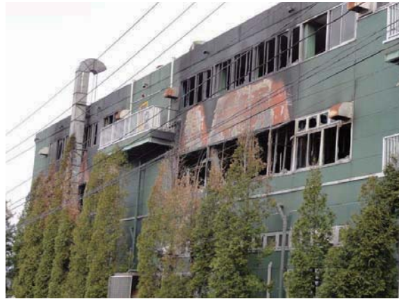
Photo 8.3-2 Fire scene at a factory building (Oushu city, Iwate prefecture)
