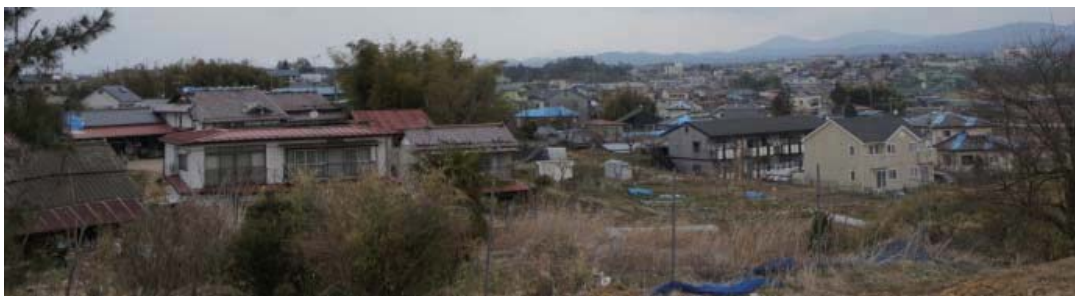
Photo 6.2-54 Damage overview from the east of Minami-machi (Many roofs covered with blue vinyl sheet)
