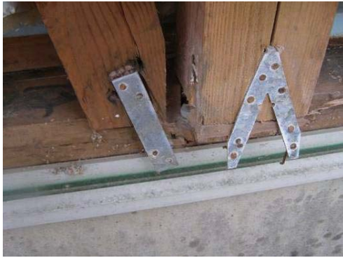
Photo 6.2-59 Metal fastener at the end of column and brace
