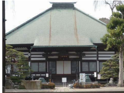
Photo 6.2-51 No damage on main hall of temple
