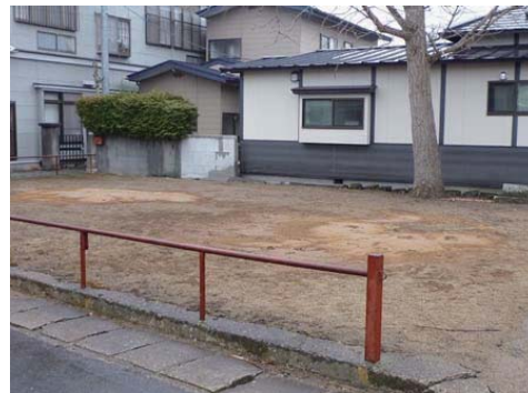
Photo 6.2-2 Sand boil due to liquefaction
