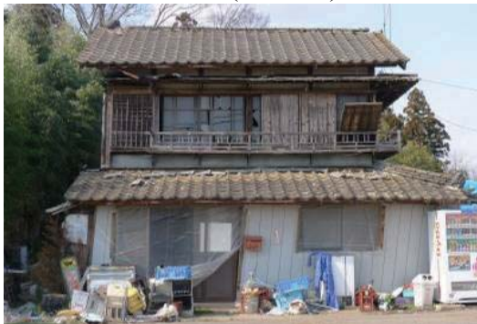
Photo 6.2-74 Damaged house with store (Kadobe)
