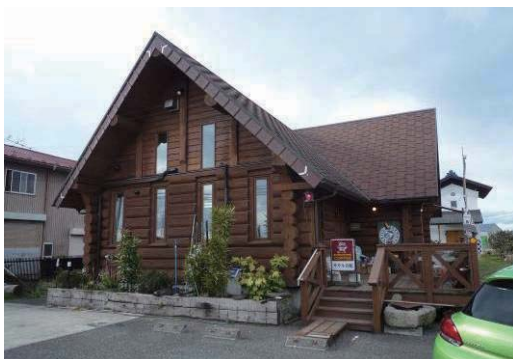
Photo 6.2-27 Log house without damage
