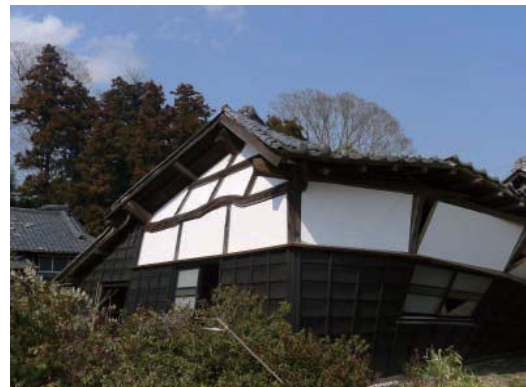
Photo 6.2-73 Tilted nagayamon gate (Kadobe)
