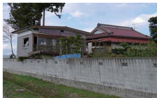
Photo 6.2-24 Collapsed wood house
