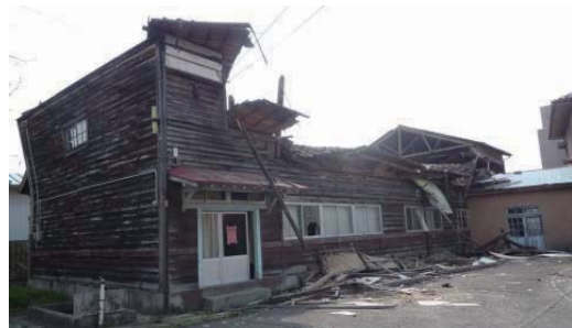
Photo 6.2-18 School building whose 2 nd story collapsed
