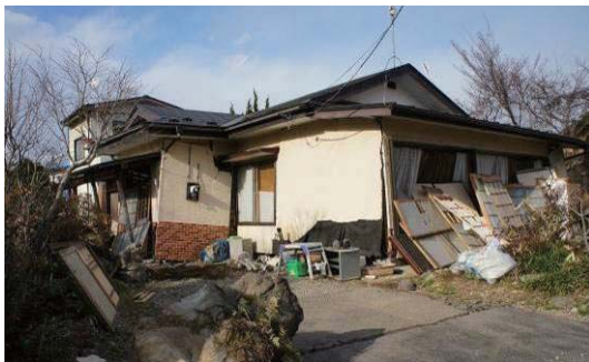
Photo 6.2-63 Wood house with large story drift
