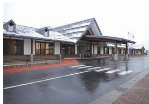
Photo 6.2-10 Kurikoma Branch office (Glulam frame structure)
