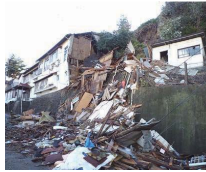
Photo 6.2-42 Collapse of Japanese-style hotel (Mukaiyama)
