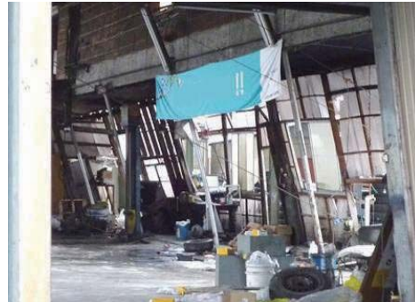
Photo 6.2-6 Inside of the building shown in Photo 6.2-5
