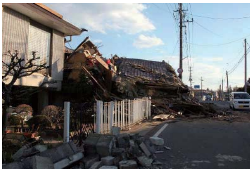
Photo 6.2-52 Collapsed wood house at Minami-machi (From Sukagawa city website)
