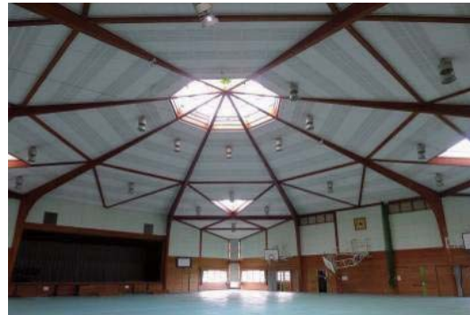
Photo 6.2-77 Inside of the gymnasium
