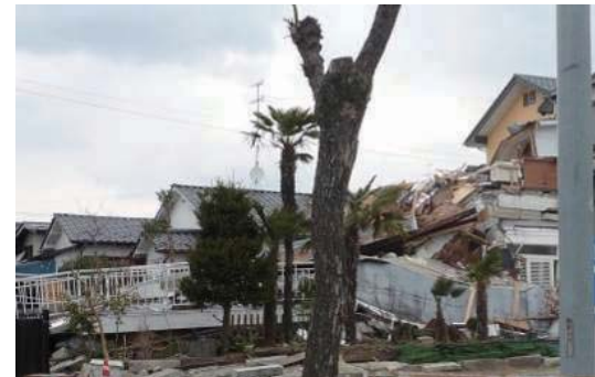
Photo 6.2-53 Collapsed building (Unknown structure type)
