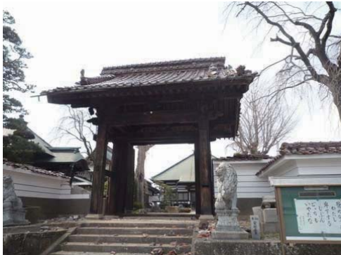
Photo 6.2-50 Minor damage of temple gate
