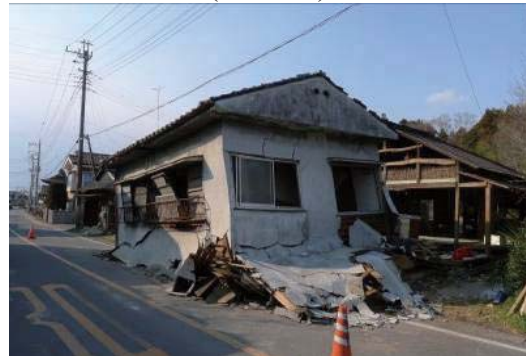
Photo 6.2-75 Collapsed house (Urizura)
