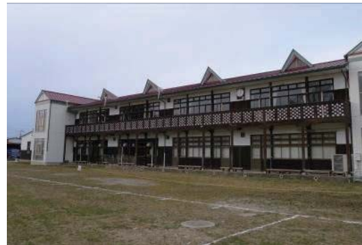
Photo 6.2-79 Wood school building
