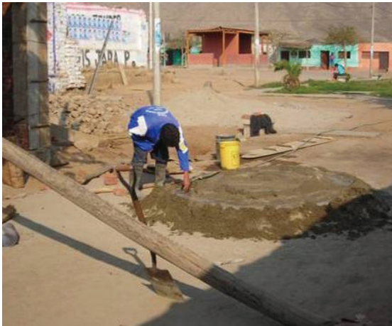
Photo.12. Pouring the concrete on the ground in Caral
