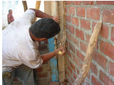
stuffing up the crack of frameworks with paper of cement
