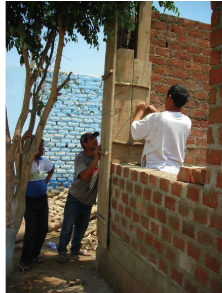
Photo.9. Reinforced Frame in Caral
