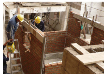
Lintel and Frame Works
