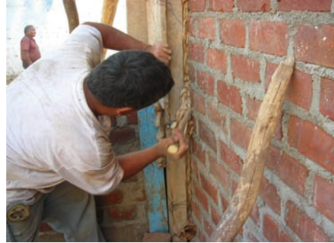
Photo.14. stuffing up the crack of frameworks with paper of cement bag in Caral
