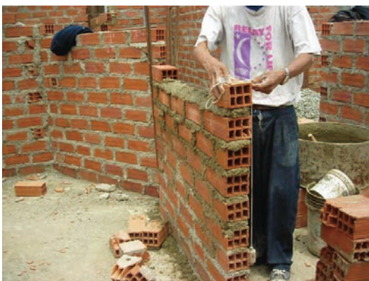
Photo.7. Picture of Neat Laying Work in Villa Salvador
