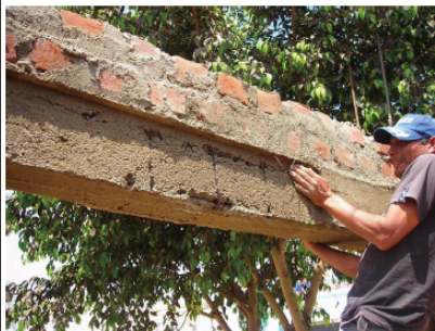
Supplement concrete subsequently
