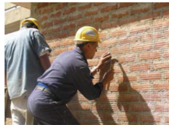
Wire Mesh Work
