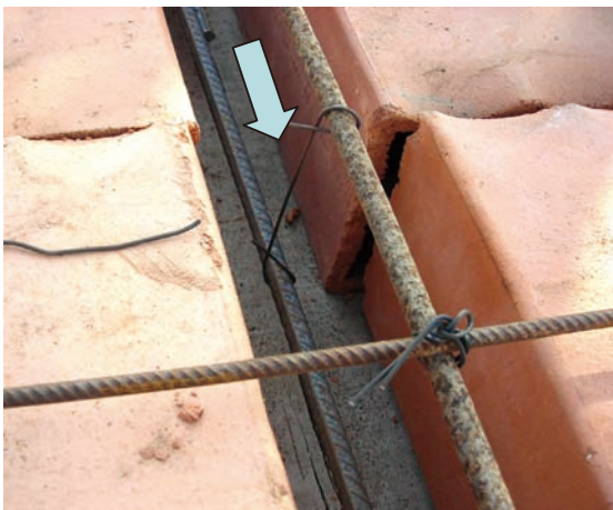
Photo.10. Using steel bar support in Villa Salvador
