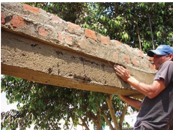
Photo.13. Supplement concrete subsequently in Caral
