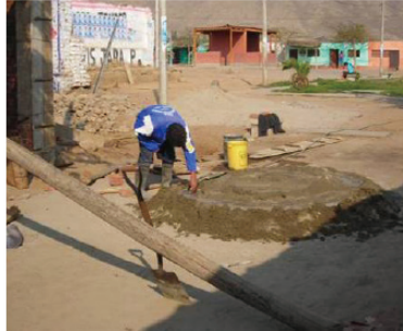
mixture concrete on the ground
