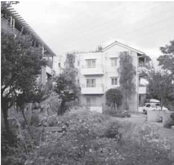
Fig. 25 Example of residential area where garden trees and green walls are used for solar shading
