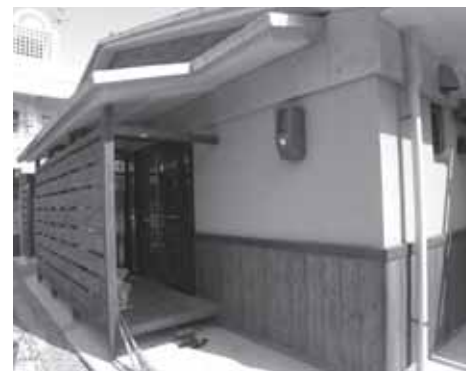
(B) Type of louver that increases the solar shading effect and keeps the louver thin
