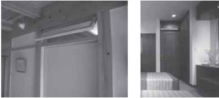
Fig. 4 Example of transom windows (effective opening area: approx. 0.1 m 2 )
