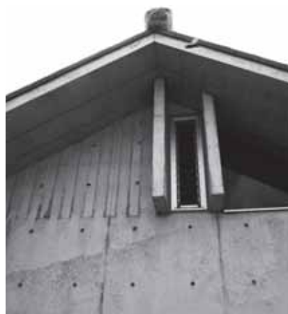
Fig. 11 Side walls installed on high window in the transverse wall
