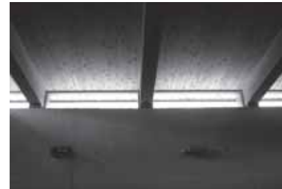
Fig. 6 Daylight guiding using reflection on ground, back of eaves and ceiling by means of amahaji
