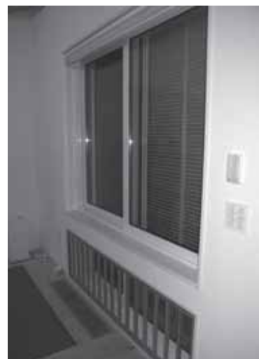
Fig. 2 Example of secured open area with security considerations Combination of a waist-level window and a small floor-level window. A wooden window bar is installed for the small floor-level window (double sliding window).
