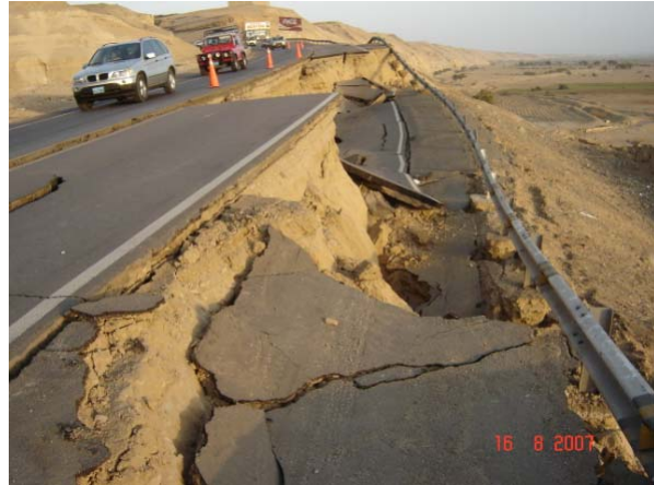
Photo 2: Cracks and subsidences of roads where traffics were restricted
