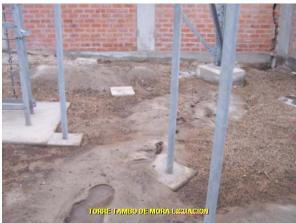
Photo 4: Damages due to liquefaction in Torre Tambo De Mora Licuaction. Many people crowded along the highway for water and food
