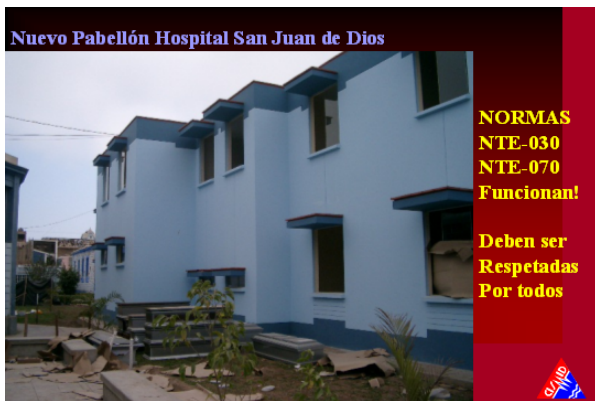
Hospital C (new building with no damage)
