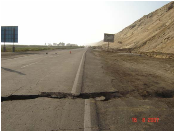
Photo 2: Cracks and subsidences of roads where traffics were restricted
