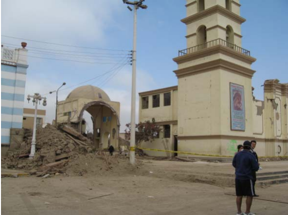
Photo 6: Damage of Church
