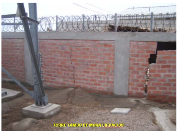
Photo 4: Damages due to liquefaction in Torre Tambo De Mora Licuaction. Many people crowded along the highway for water and food
